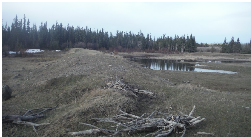
Figure 4: Decommissioned Sword Creek Reservoir #2 dam, view looking west with flow from right to left.
